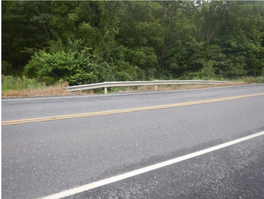
Photo No. 7 - West guide rail
