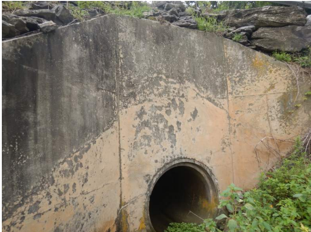
Photo No. 1 - Upstream elevation
