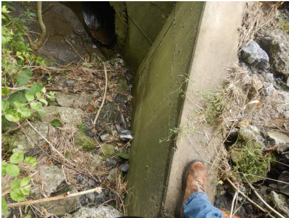
Photo No. 8 - Typical wingwall
