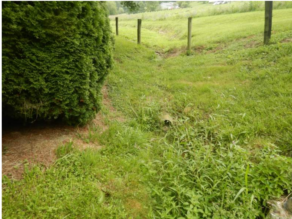
Photo No. 13 - Upstream channel (concrete pipe)
