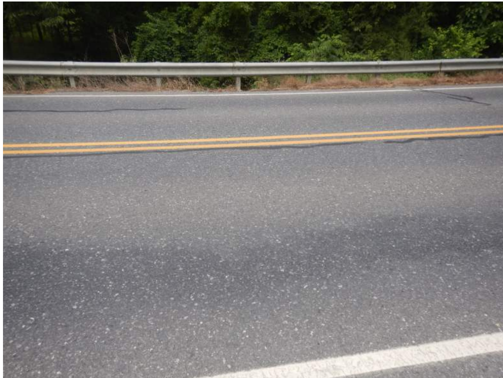
Photo No. 5 - Typical deck
