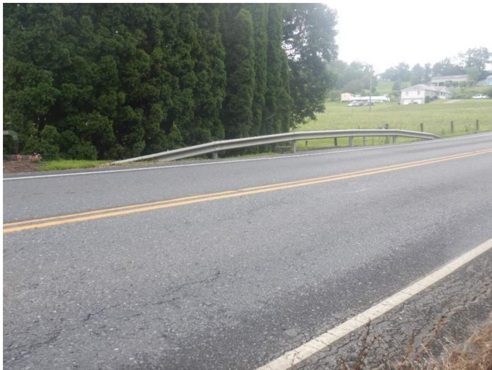
Photo No. 6 - East guide rail
