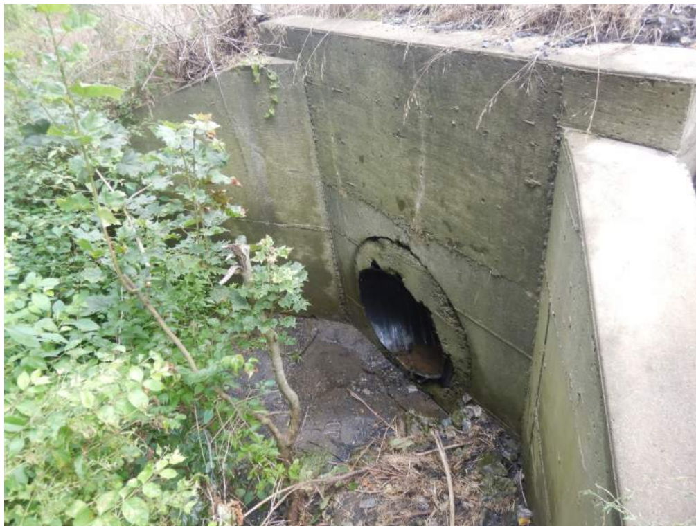
Photo No. 2 - Downstream elevation
