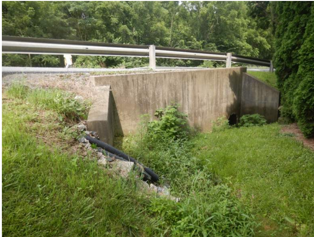
Photo No. 1 - Upstream elevation
