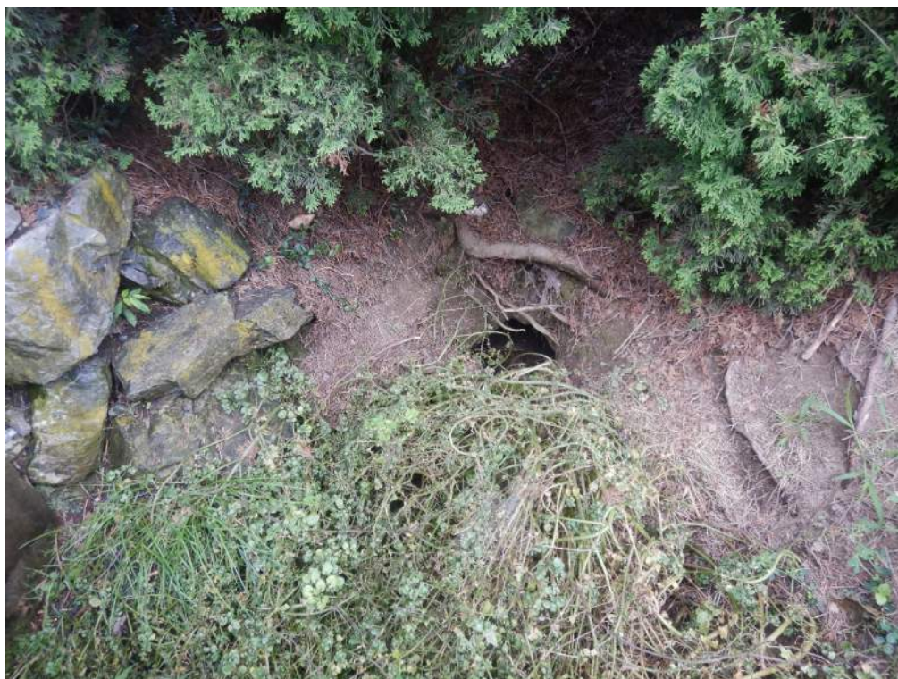
Photo No. 14 - Upstream channel (creek)
