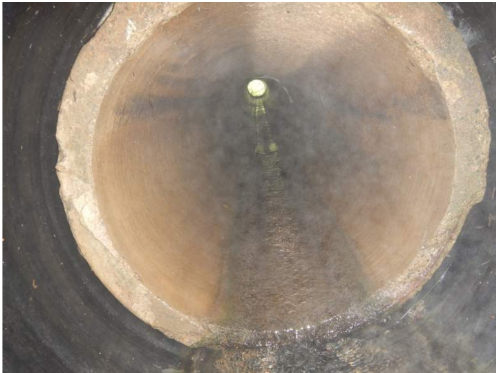
Photo No. 10 - Downstream pipe transition
