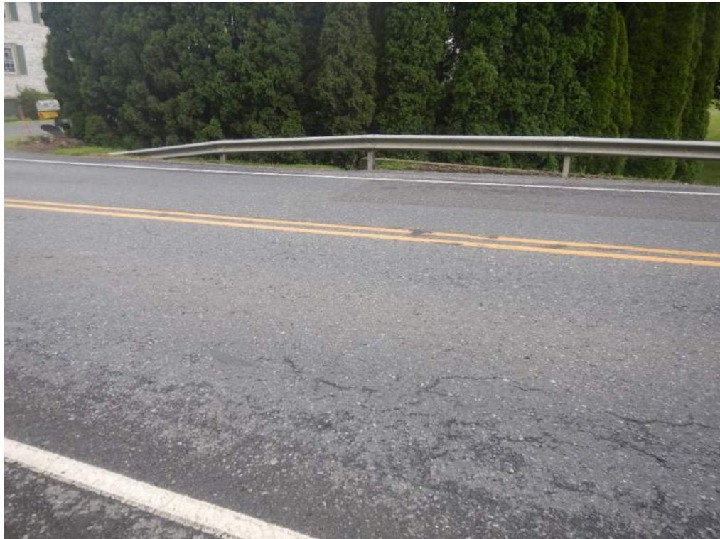
Photo No. 5 - Typical deck
