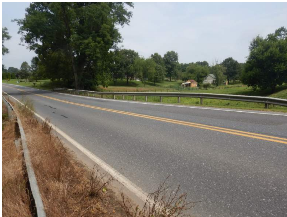
Photo No. 6 - East guide rail
