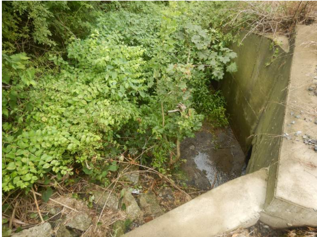
Photo No. 12 - Downstream channel
