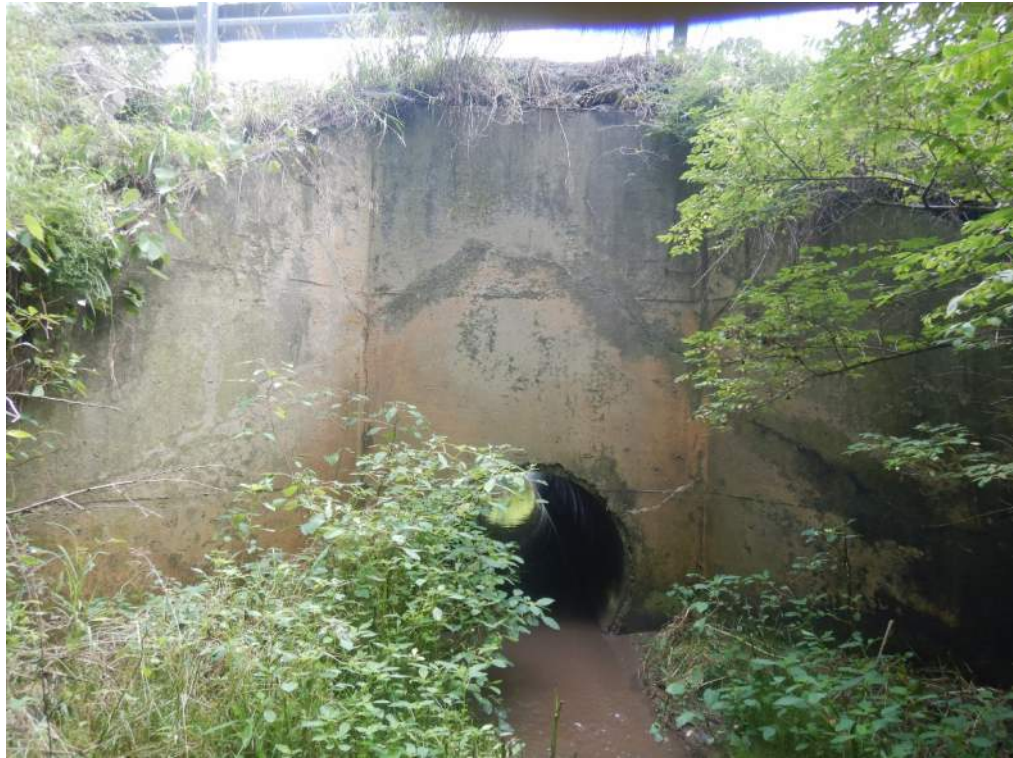
Photo No. 2 - Downstream elevation
